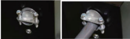
Figure 11: Installing cable fitting to heater
